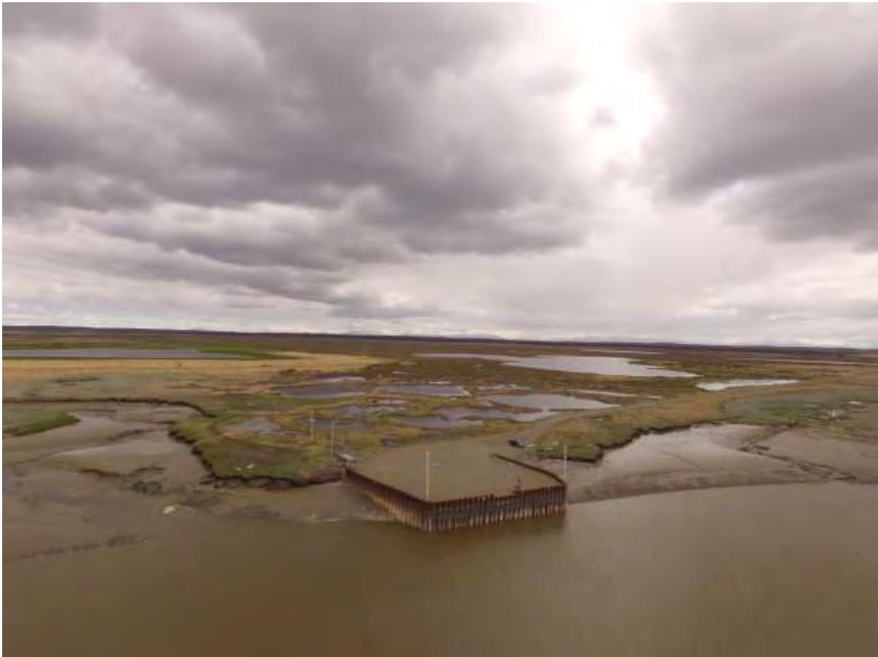
**Figure 8.** Unmanned aerial vehicle (UAV) photograph of the Pilot Point bulkhead taken during summer field work. The bulkhead is currently being damaged by erosion and flooding. This infrastructure is critical to the commercial salmon fishery including the planning for a new seafood processing plant. Data provided through this project has contributed towards developing mitigation strategies for its possible fortification and/or replacement.
